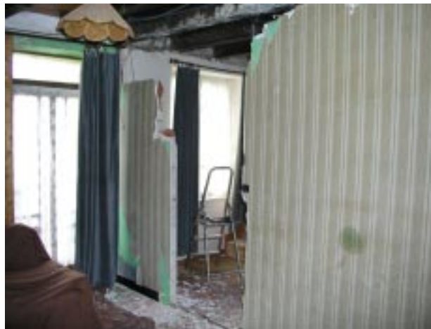
The start of the demolition
